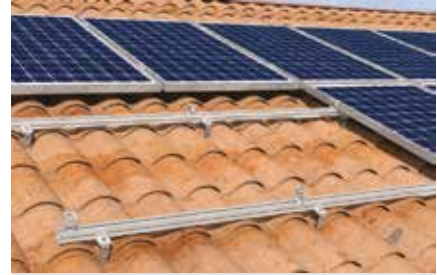
Detail: clamps position
