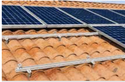
Pitched roof with tiles
